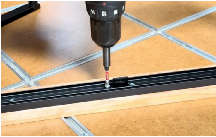
Figure 11 — Installing the security clip
