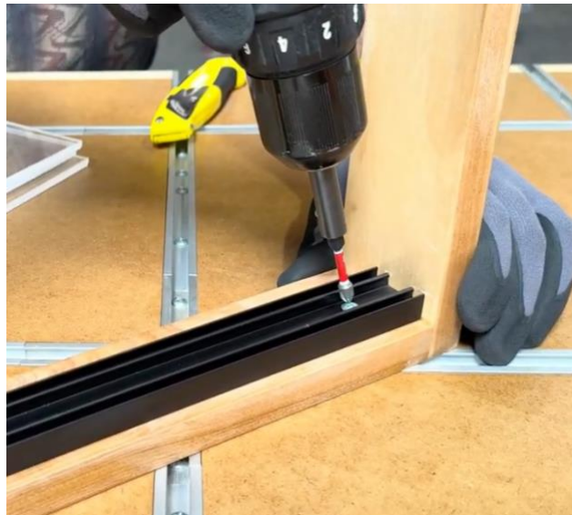
Figure 10 — Mounting the upper and lower tracks
