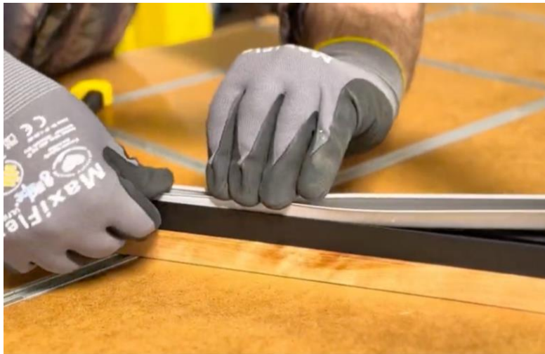
Figure 12 — Installing the deep header inserts
