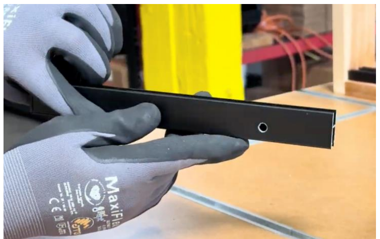
Figure 8 — Drilling the lock hole (detail)
